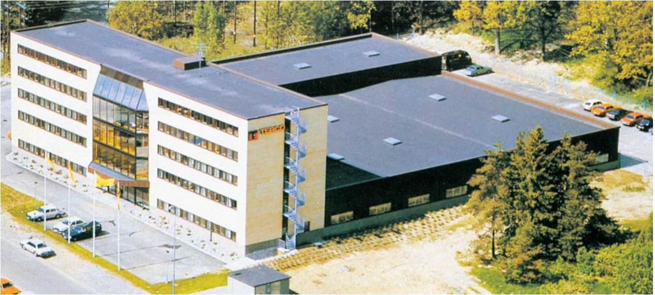
Terco headoffice and factory outside Stockholm, Sweden.
