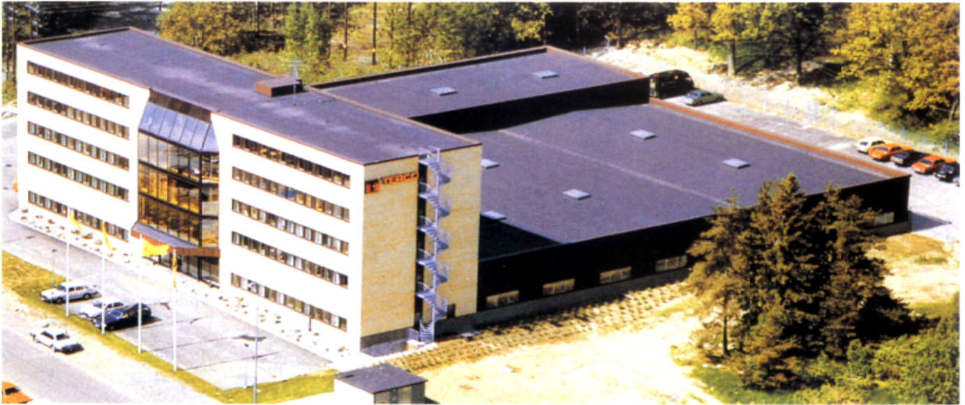
Terco headoffice and factory outside Stockholm, Sweden.
