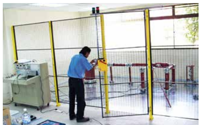
Installation of High Voltage Equipment
