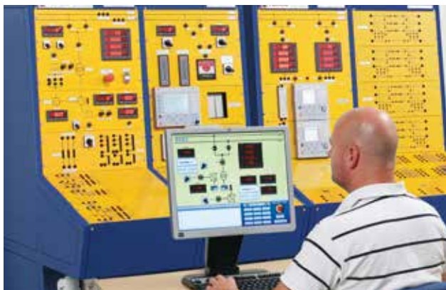
The Terco PST-SCADA system
