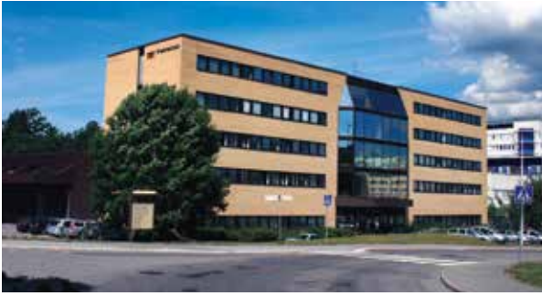
Terco headoffice and factory outside Stockholm, Sweden
