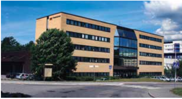
Terco headoffice and factory outside Stockholm, Sweden
