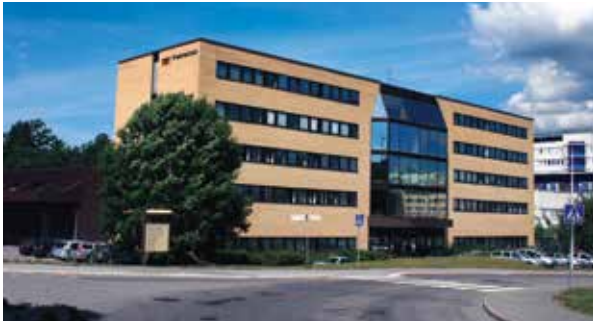
Terco headoffice and factory outside Stockholm, Sweden
